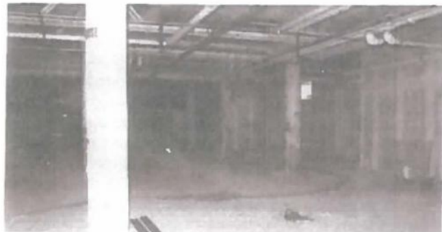
The 12th floor of the Wanamaker Building during restoration. At a rent of $16.50 per square foot, the complex litigation center pays less than it would for comparable space in the City Hall area. Judges have found the building's high ceilings ideal for the center's courtrooms.
